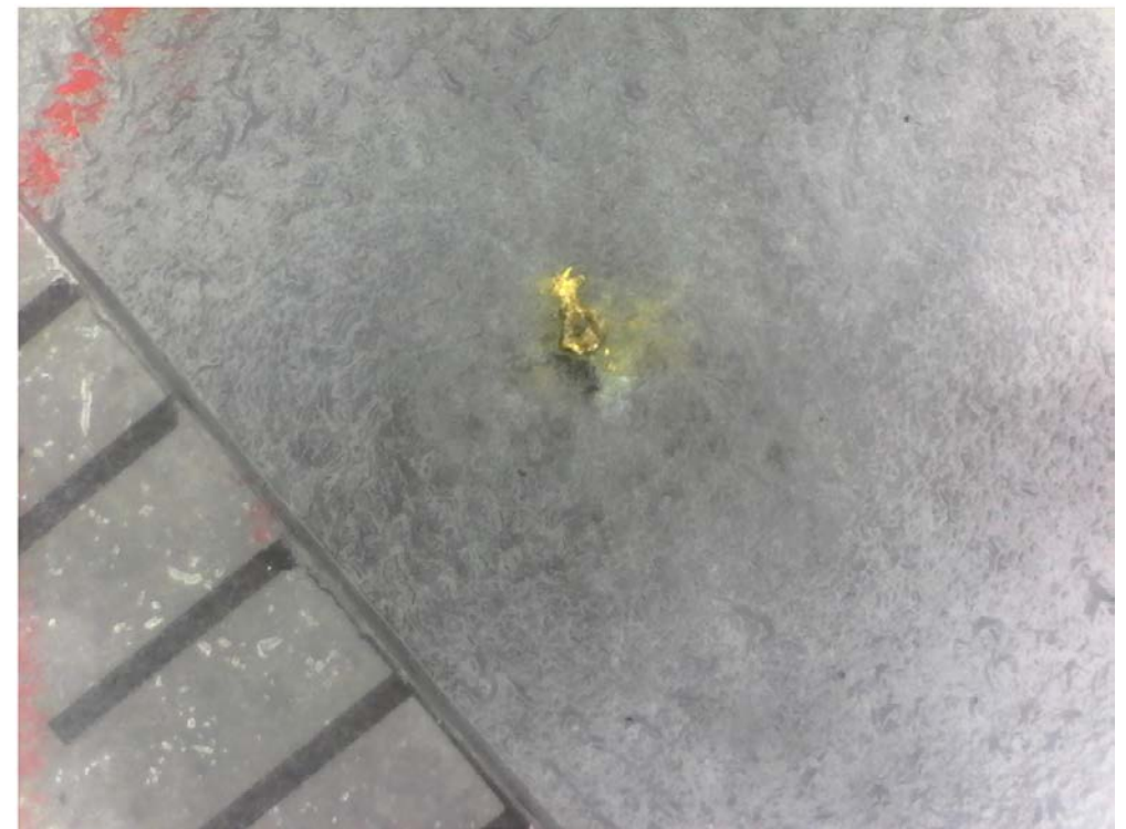
Middle Structure – 192m
