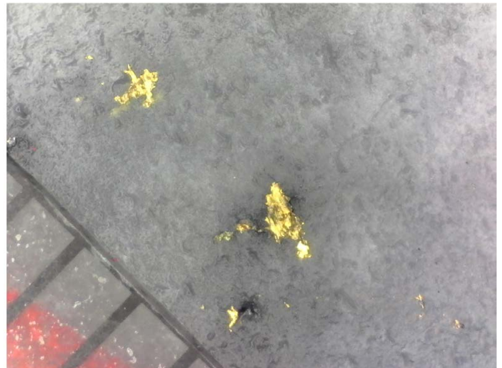
Middle Structure – 192m
