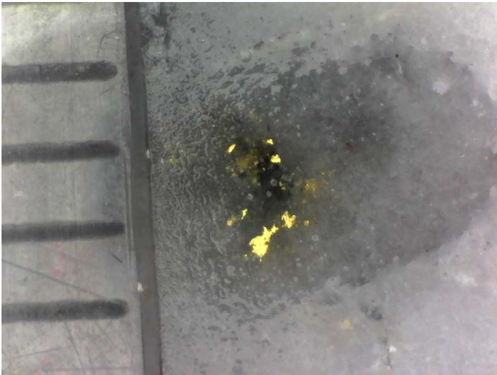
Middle Structure – 342m
