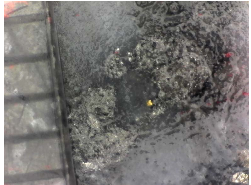
Middle Structure – 342m
